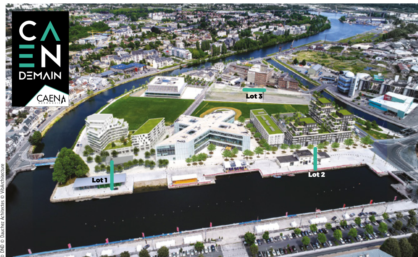
© DND © Dauchez Architectes © VibaArchitecture
